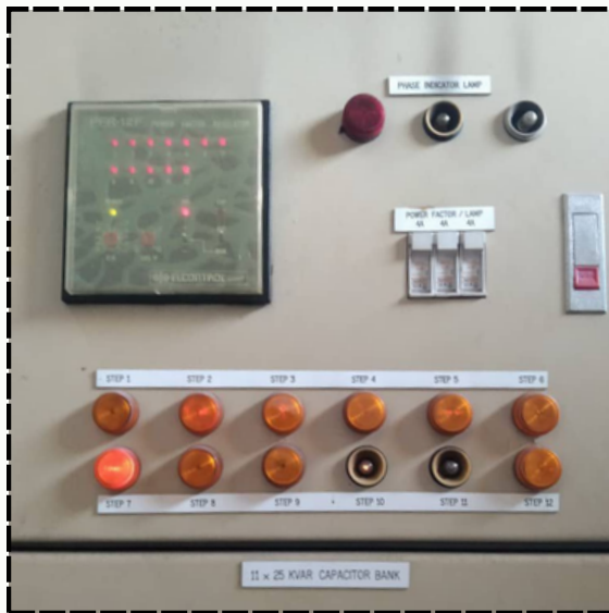
The capacitor bank is no longer working. The indicator light is not on
